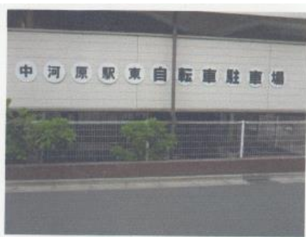
側面 (side of parking lot)
